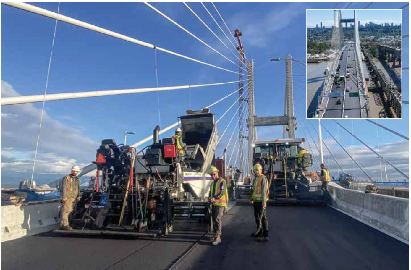
Members with BA Blacktop paving the staləwasəm Bridge.
