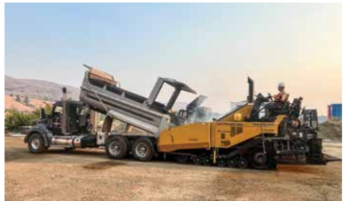
Dan McKie and Rob McKie working with Vernon Paving Ltd.
