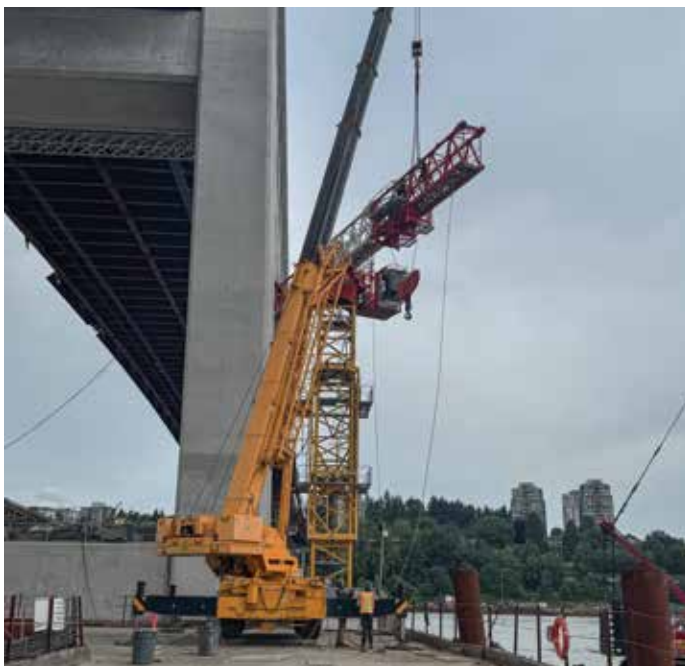
Members at Fraser River Pile and Dredge assisting with the MDT809 dismantle on the staləwəsm Bridge.
