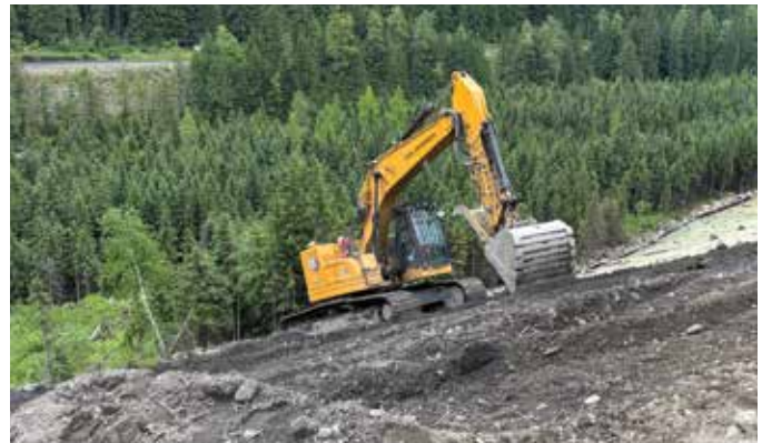
Cole Anchikoski working on the BCIB Highway 1 four-laning at Jumping Creek.
