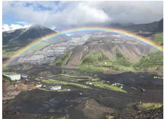
Elk Valley Resources Line Creek Operations - Mine operations and maintenance building (left) and coal dump (right).
