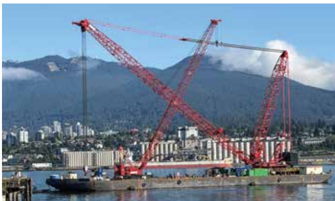
Dynamic Installations new 900 T ring crane, The Dynamic Berzerker under tow to it's first job.
