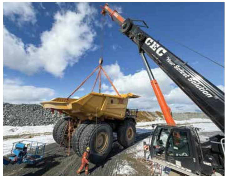
Cutting Edge Crane installing a dump box on a haul truck.
