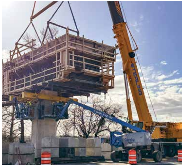
Sterling Crane working at the Surrey-Langley SkyTrain Project.
