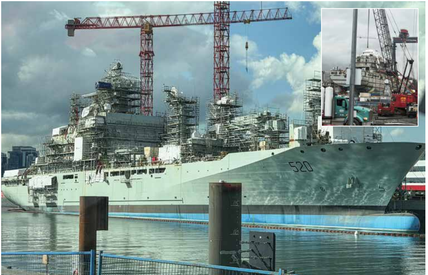
Badger Daylighting and Fraser River Pile and Dredge at Seaspan shipyards in North Vancouver working together on building up Canada’s defences and strengthening our sovereignty.
