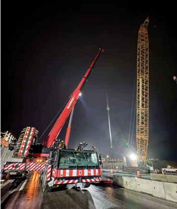
Tyler Buerge operating Mammoet's LTM 1400 performing girder install with KEA on Highway 1 at 264 th overpass.
