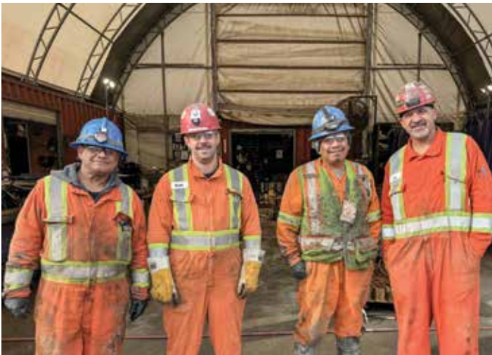
Members at Eagle Mountain-Woodfibre Gas Pipeline Project.
