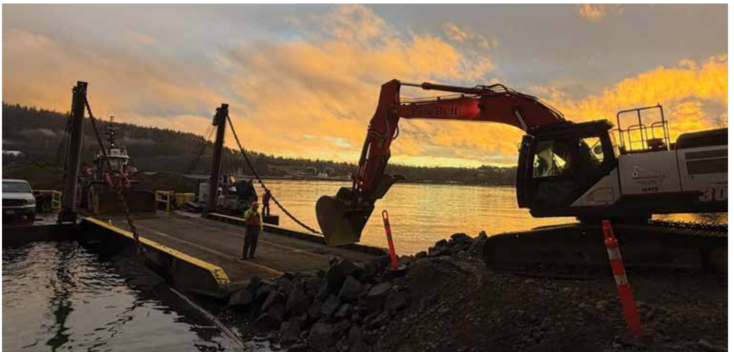
Upland Contracting working at Cates Park in North Vancouver.
