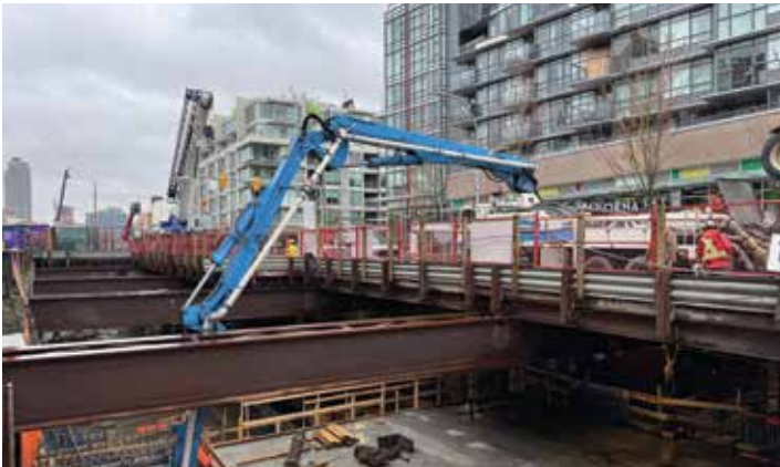
Gastaldo Concrete pumping concrete in tunnel on the Broadway Subway line at Arbutus Street.
