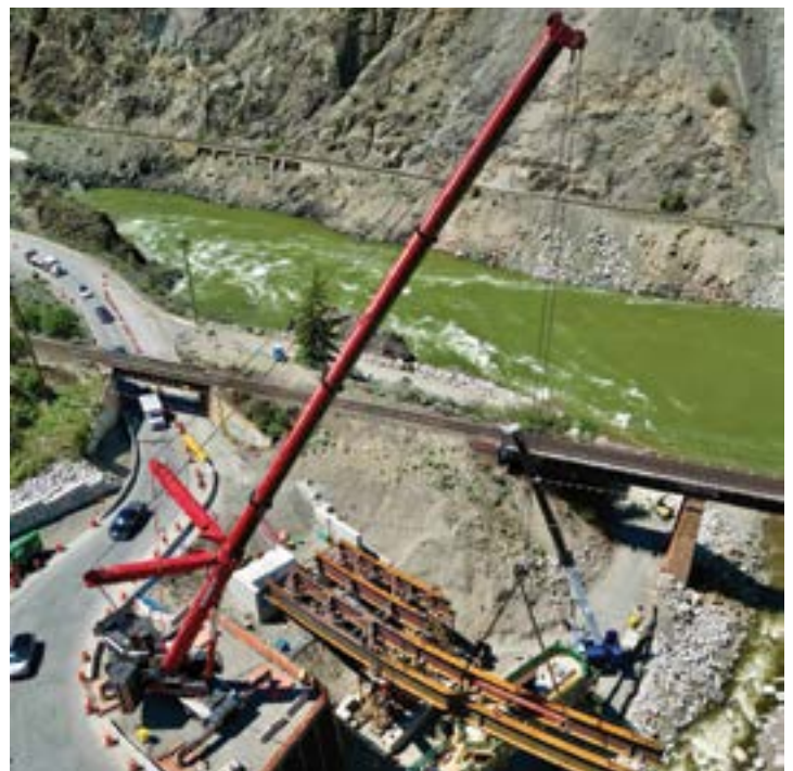
Members Tyler Buerge and Matt Gillis working on the Nicomen Bridge.
