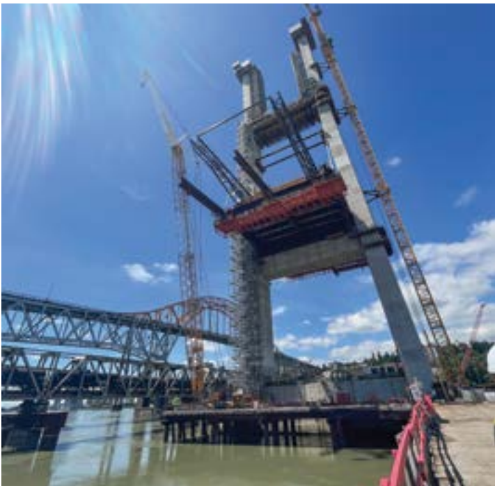
Pattullo Bridge Replacement Project.
