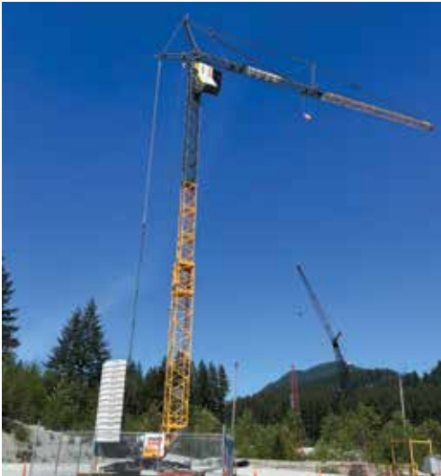
Liebherr 81K Self-Erect Tower Crane at the IUOETA training site. Thanks to Morrow Crane and their crew in assisting us with the installation of this crane.
