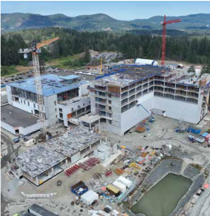
Drone shot of the Cowichan District Hospital Replacement Project. Image courtesy of Island Health and EllisDon
