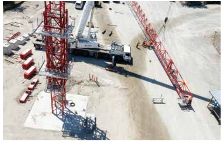
Members from both RKM and Oxford Builders working together assembling the Potain MDT 219.
