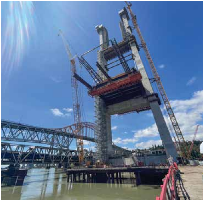
Pattullo Bridge Replacement Project.
