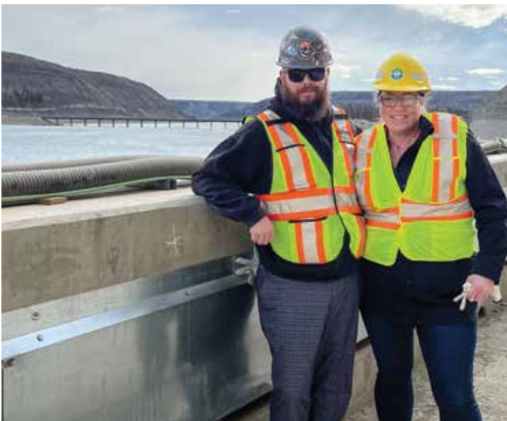
Business Representative Konrad Tarry and BC Building Trades Executive Director Brynn Bourke on a recent visit to the Site C Dam.
