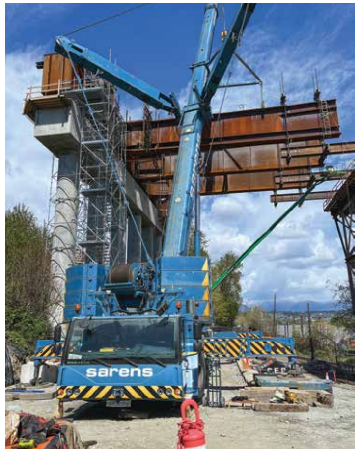
Sarens crane working on the Pattullo Bridge Replacement Project.
