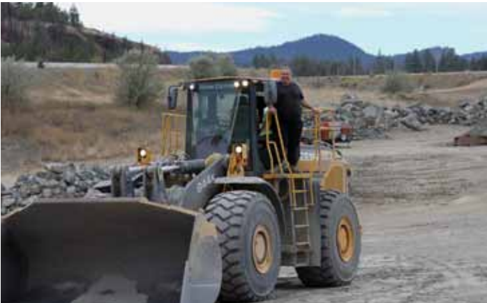
Brother Don Smith working with the Emil Anderson portable paving plant at Pritchard.
